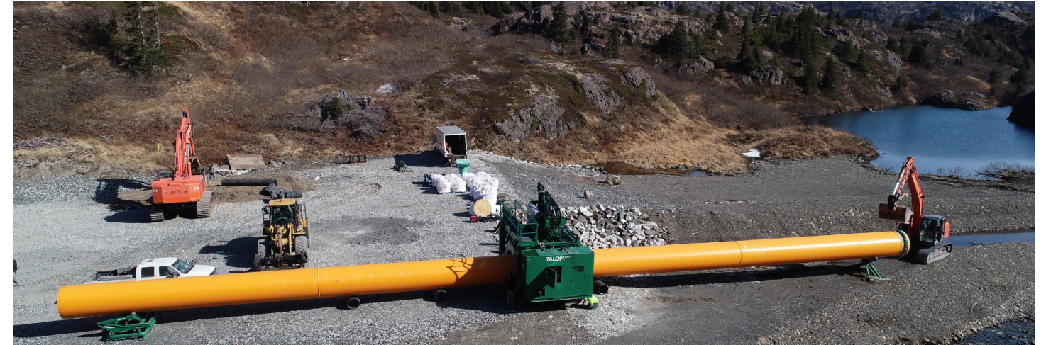
Contractors at the West Fork Upper Battle Creek Diversion project site fuse two sections of high-density polyethylene pipe using the world's largest fusion welding machine, which was brought in from the Lower-48.
